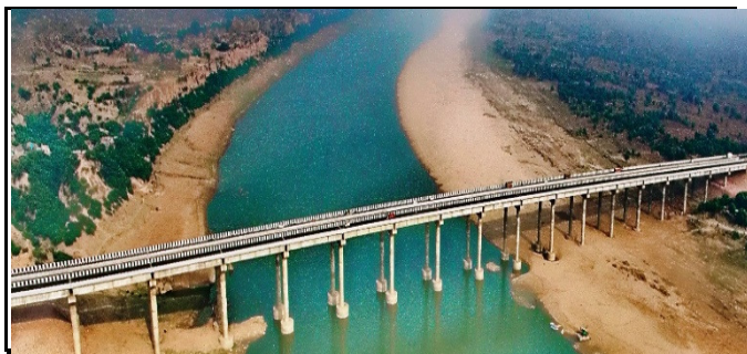
Fig. 1. Bridge over river Chambal at Dholpur
